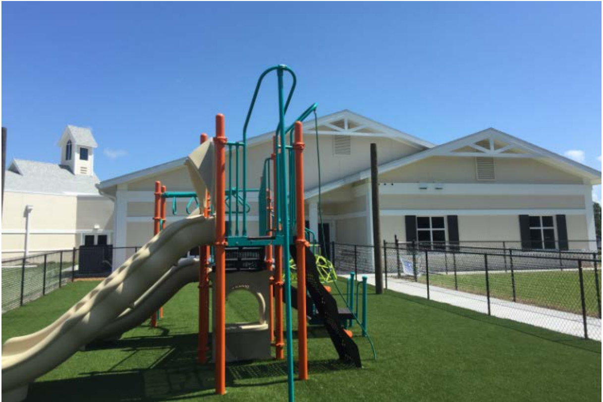
ABOVE: The Children's Wing at Christ Church Vero Beach features classrooms, a kid's Chapel and an outdoor playground. Located at the corner of State Road 60 and 6 th Ave. in Vero Beach, a dedication and consecration service is planned for 10 a.m. Sunday Oct. 8.
